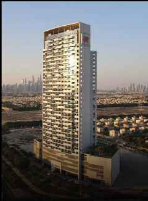
Al Jawahara Tower JVT, Dubai
