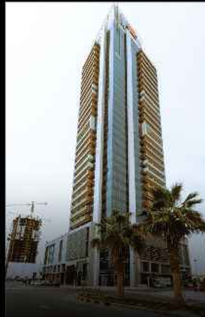
Al Manarah Tower JVT Dubai
